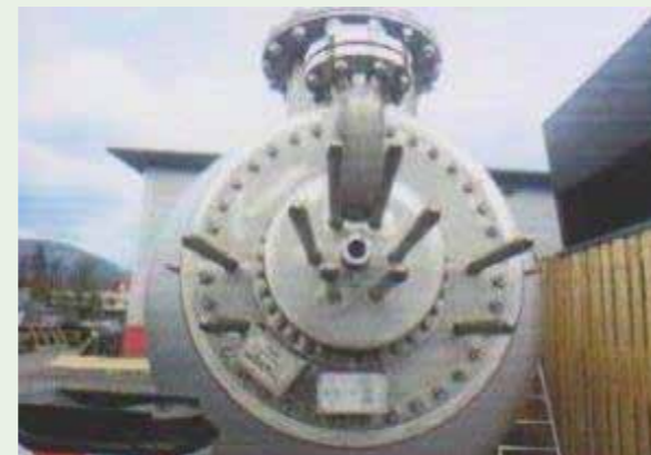
↑ Halogenated Hydrocarbon Thermal Oxidizer
