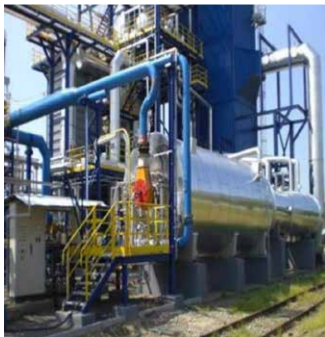
^ Spent sulphuric Acid Regeneration
