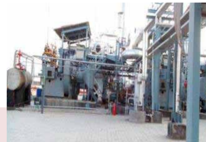
▲ Plant: HSD / LPG fired solutions
