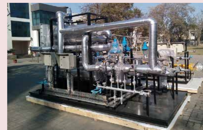
^ Fuel Conditioning and Control Station
