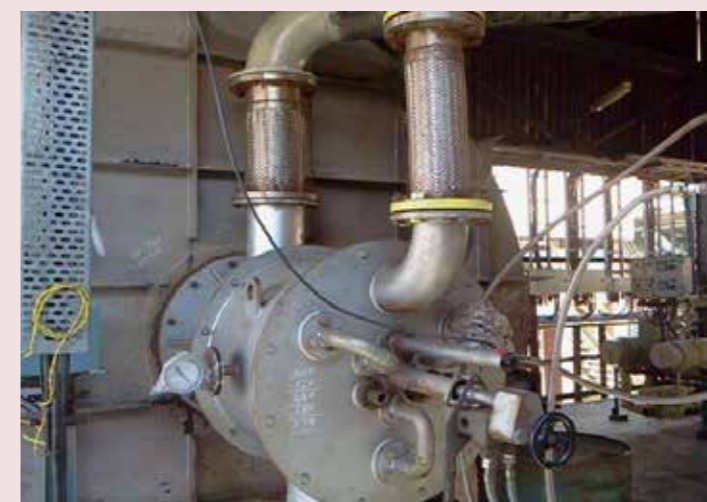
^ Tri fuel Fired Solution for Calciner Klin Hydrogen Gas + Producer Gas + HFO
